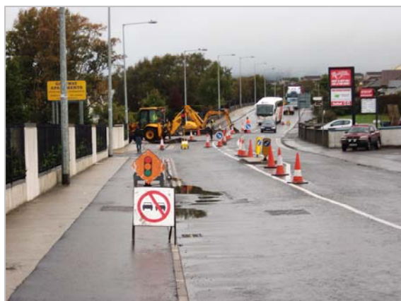
Water Conservation – Stage 3 Works Phase 1 (Sligo City) - Site Investigation Contract
