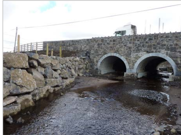
Installation of the new concrete arch extension system The completed job, N17 near Curry
