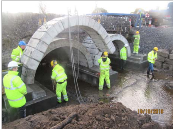
Installation of the new concrete arch extension system The completed job, N17 near Curry
